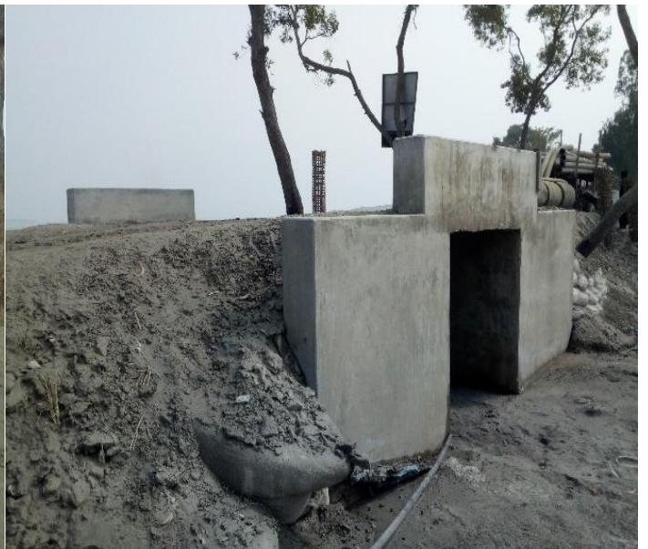
Box culvert was constructed in joint initiative like LoGIC at Ranigonj,Chilmari
