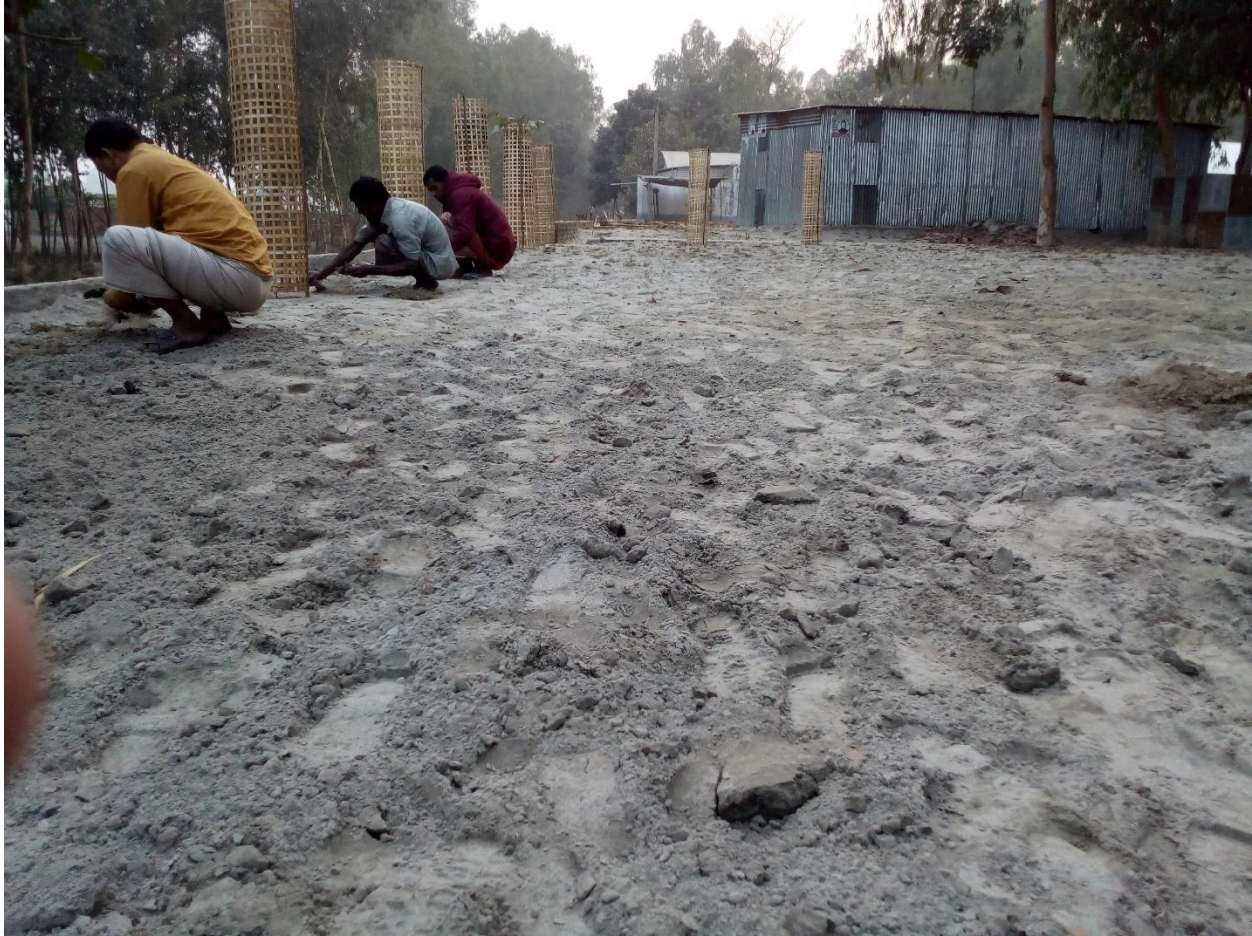
Community Ground (temporary shelter) raised at Jorghach, Ramna, Chilmari
